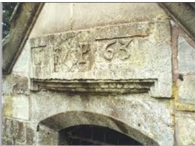
The lintel over the entrance to the well
