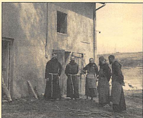
Building work on the vineyard house
