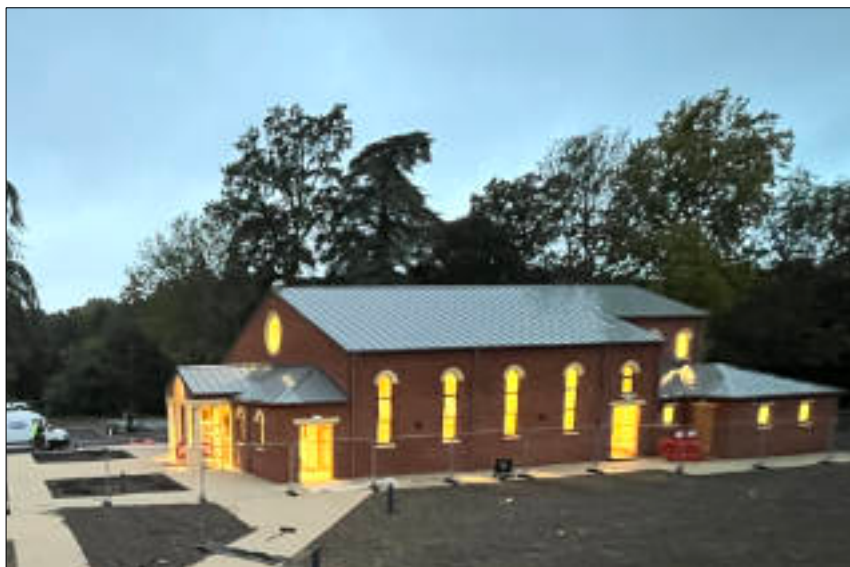
Working around the clock to get St. Michael Archangel Church ready.
