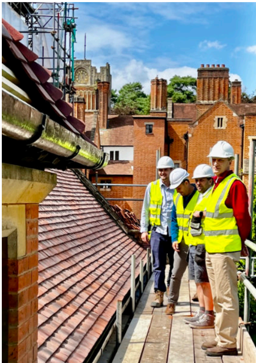
Meanwhile, Mr. Richard Squire inspects the re-roofing of Holy Cross, Woking.
