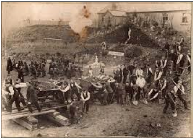
Workers on the construction site
